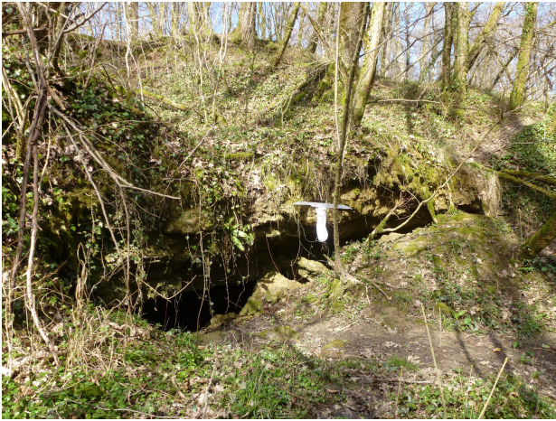
Figure 3. Entrance to the Agouti 1 underground quarry. The entrance is blocked by the soil from the erosion of the hill since the quarry was closed.
